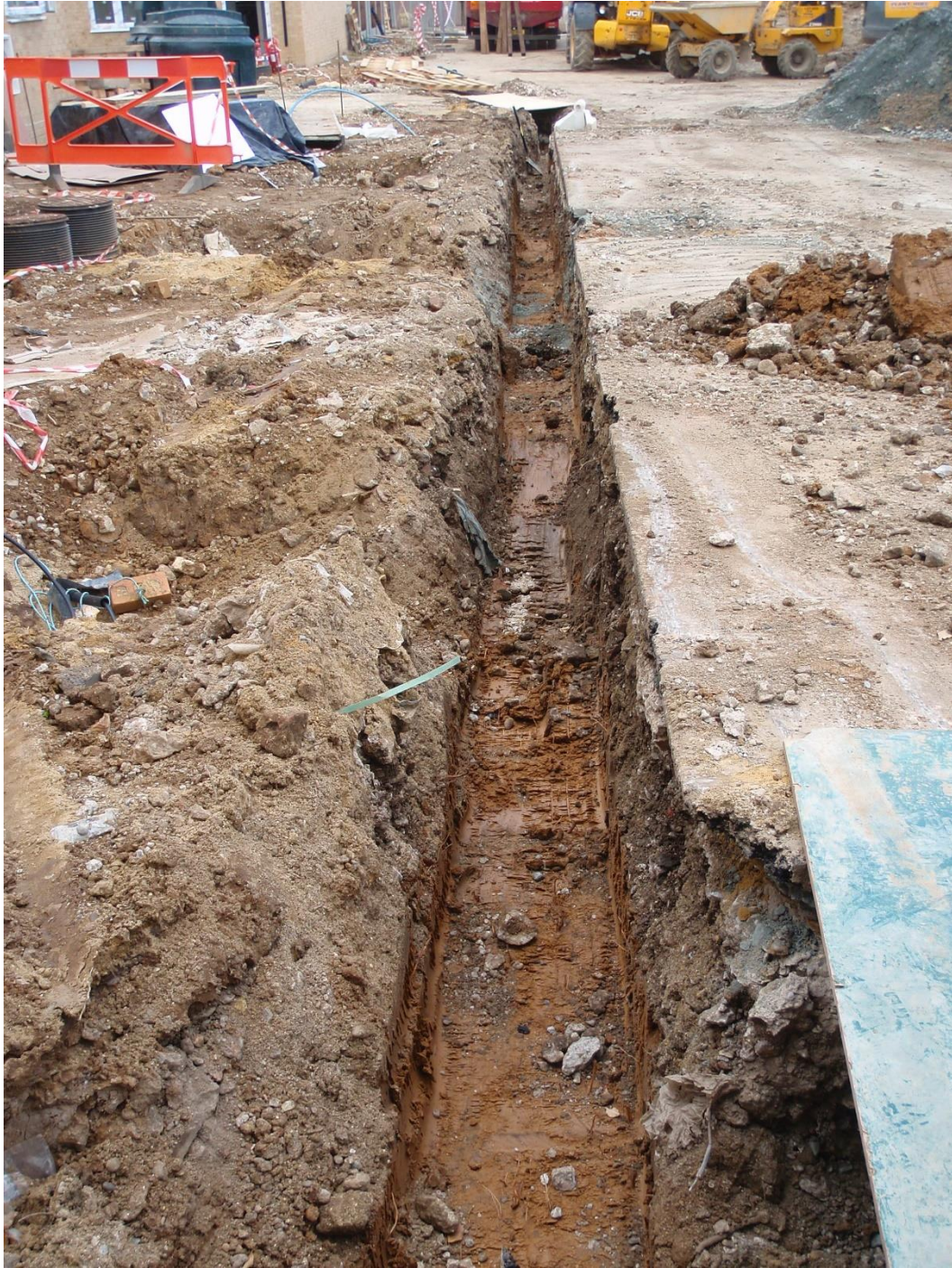
Plate 7 Archaeological monitoring carried out during the excavation of service trenches
